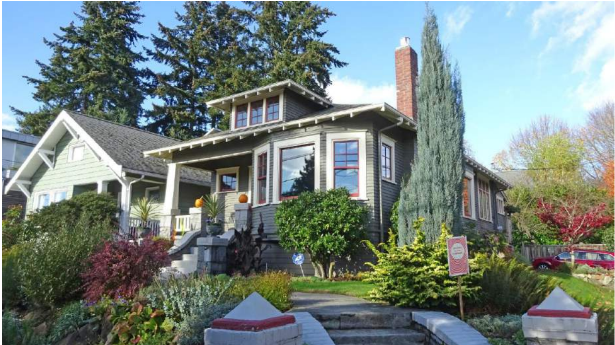
WA_King County_Wallingford-Meridian_Streetcar_HD_0027. 2120 N 46th Street, looking northwest.
