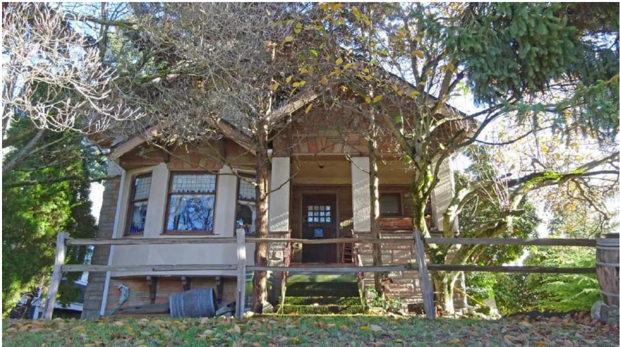
WA_King County_Wallingford-Meridian_Streetcar_HD_0026. 4604 Meridian Avenue N, looking east.
