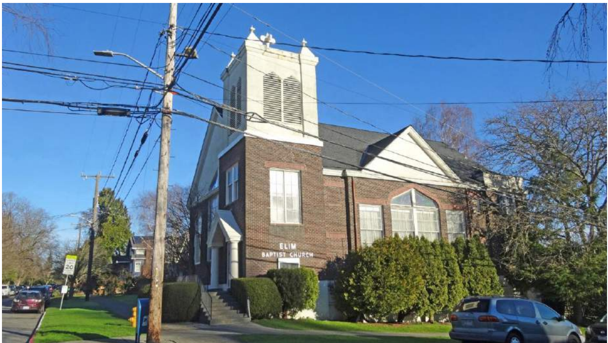
WA_King County_Wallingford-Meridian_Streetcar_HD_0028. Elim Baptist Church, looking north.
