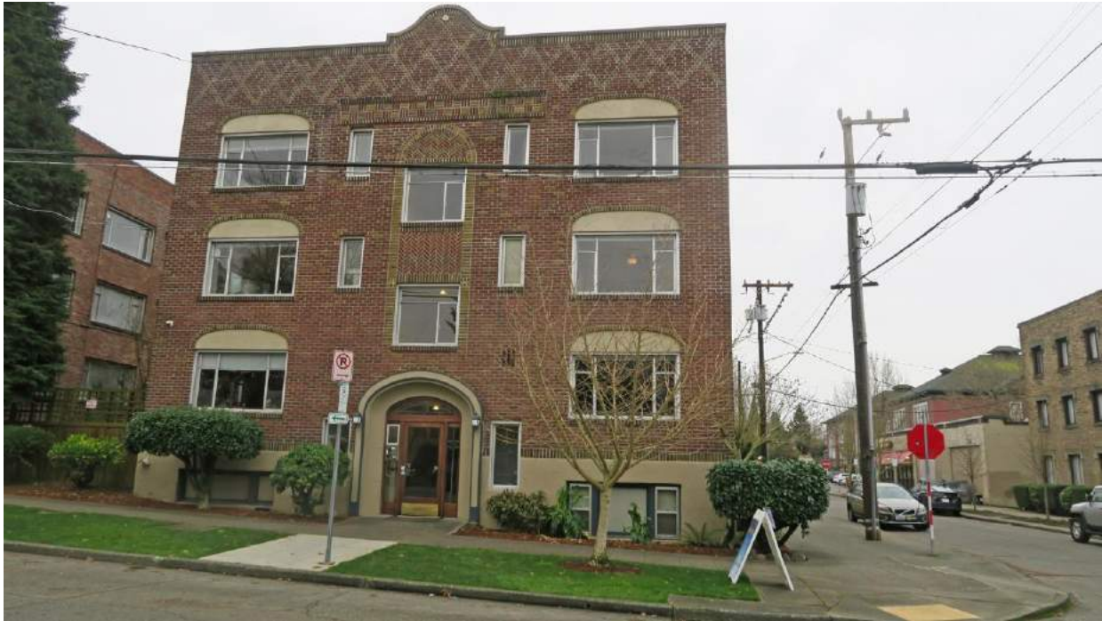
WA_King County_Wallingford-Meridian_Streetcar_HD_0017. 1903 N 46th Street, looking south.
