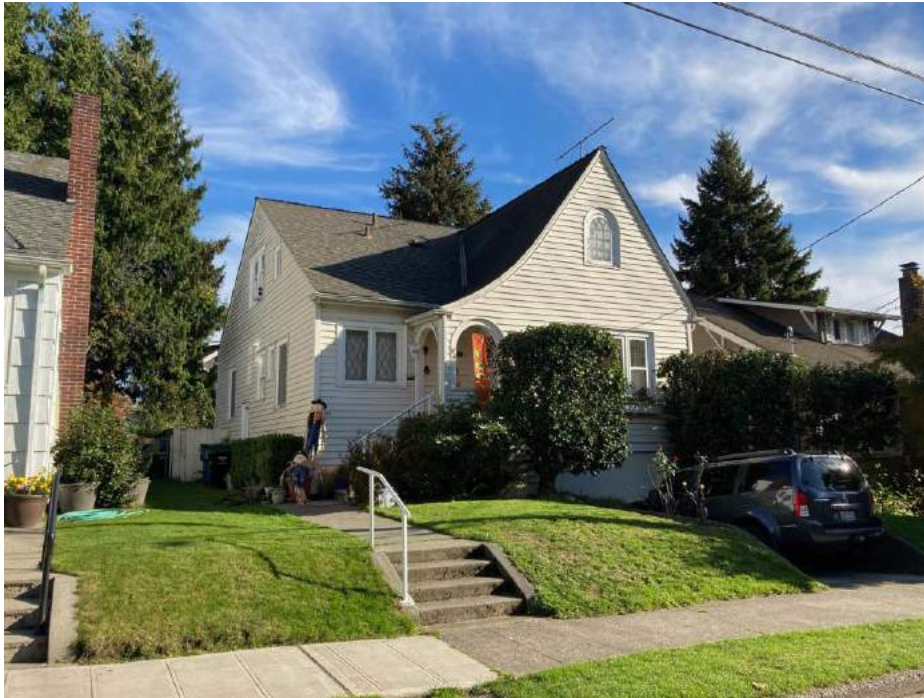
WA_King County_Wallingford-Meridian_Streetcar_HD_0037. 4626 1st Avenue NE, looking southeast.
