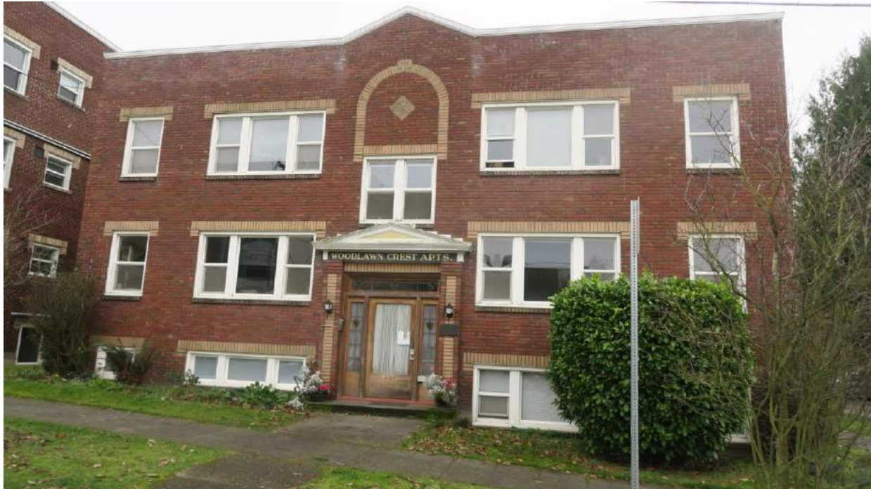
WA_King County_Wallingford-Meridian_Streetcar_HD_0007. 1603 N 46th Street, looking south.
