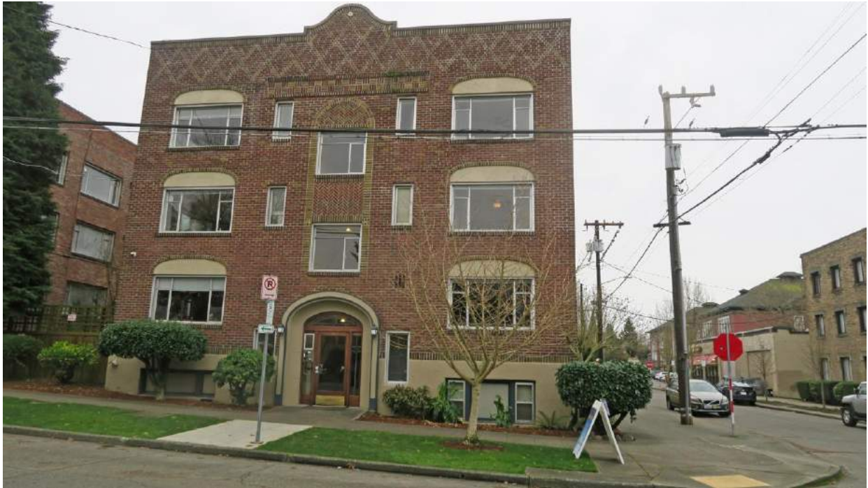
WA_King County_Wallingford-Meridian_Streetcar_HD_0017. 1903 N 46th Street, looking south.
