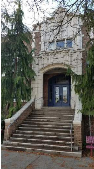
WA_King County_Wallingford-Meridian_Streetcar_HD_0011. 1703 N 49th Street, front entrance detail, looking west.
