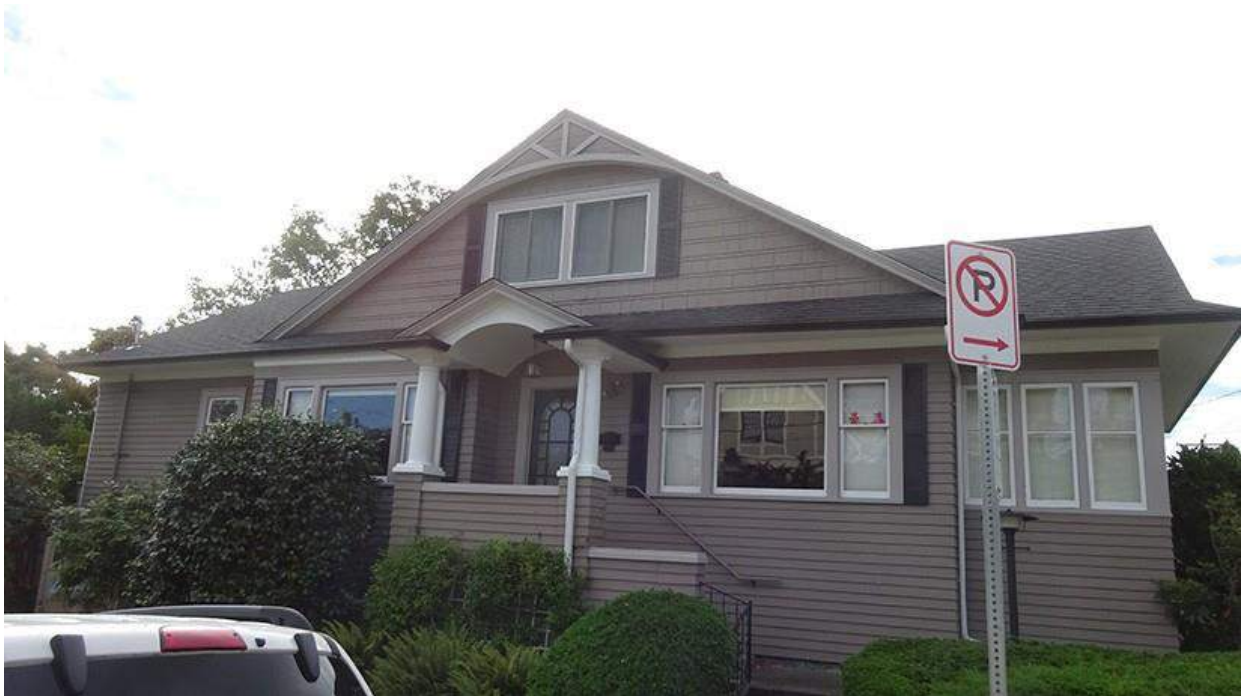
WA_King County_Wallingford-Meridian_Streetcar_HD_0044. 4558 Latona Avenue NE, looking southeast.
