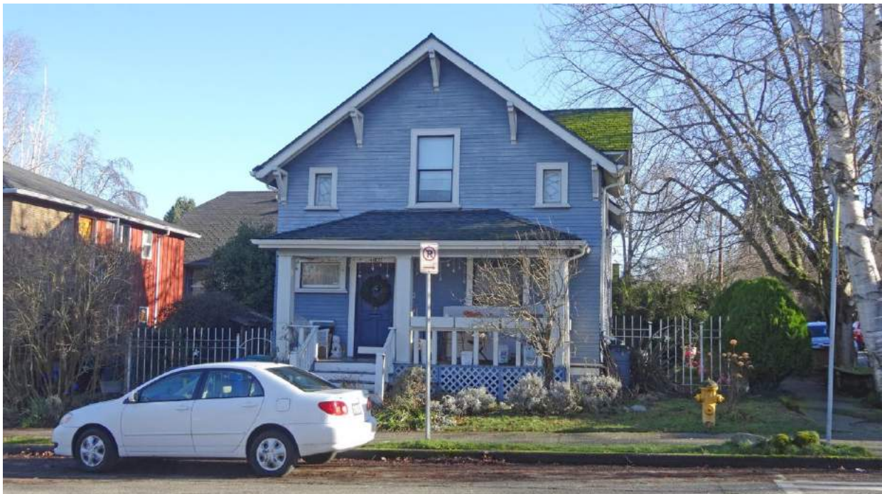
WA_King County_Wallingford-Meridian_Streetcar_HD_0002. 4802 Interlake Avenue N, looking east.
