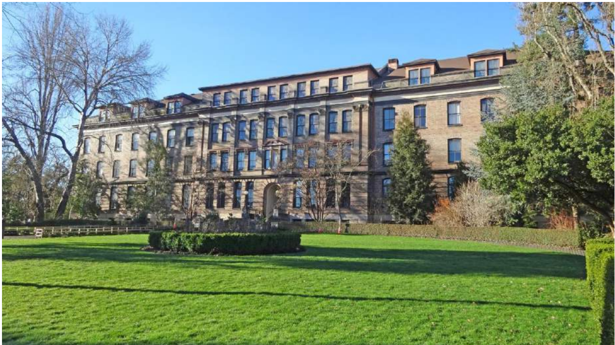
WA_King County_Wallingford-Meridian_Streetcar_HD_0056. Good Shepherd, looking southwest.
