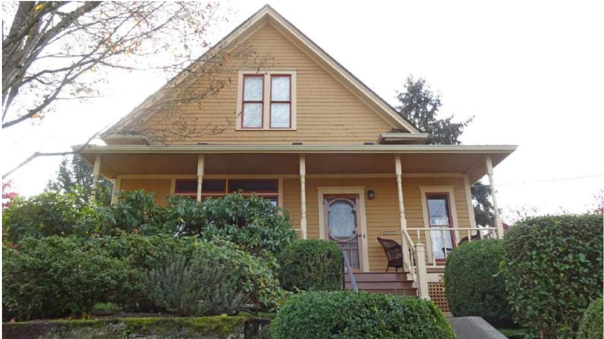
WA_King County_Wallingford-Meridian_Streetcar_HD_0005. 1603 N 48th Street, looking south.
