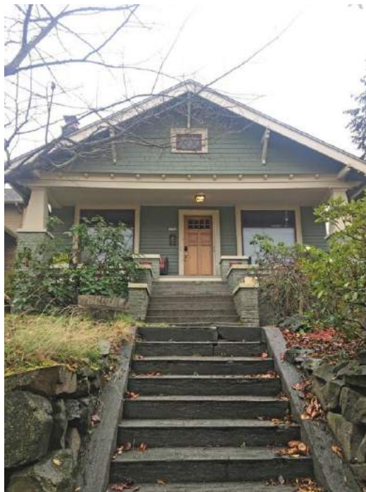
WA_King County_Wallingford-Meridian_Streetcar_HD_0010. 1711 50th Street, looking south.
