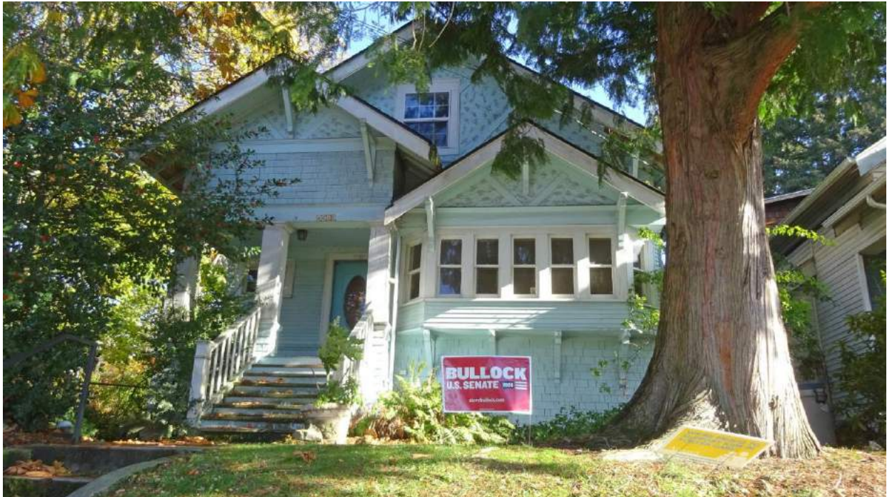
WA_King County_Wallingford-Meridian_Streetcar_HD_0025. 4616 Meridian Avenue N, looking east.
