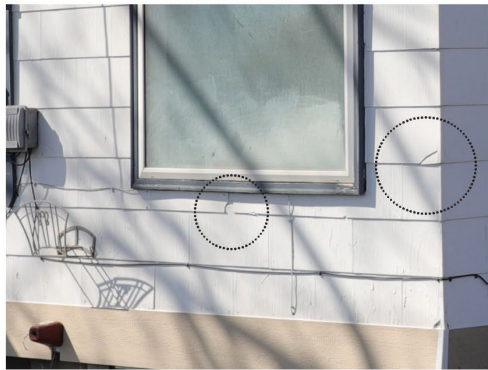
Asbestos shingles , look for thin material, and chips or broken corners.
