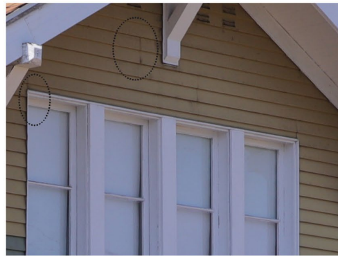
Aluminum siding , look for dents or double vertical joints, and metal trim around windows and doors locking siding ends in place.
