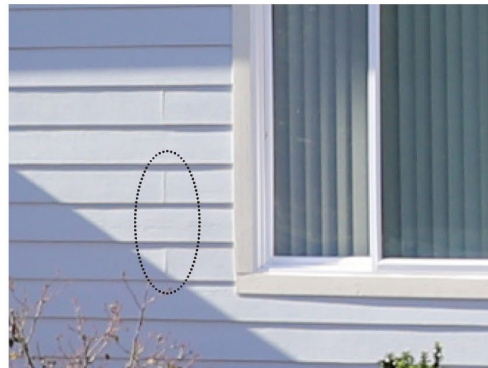
Fiber cement board , look for 1/8-inch wide joints at board ends that have been caulked, and crisp edges/textures, and corner boards to cover seams.
