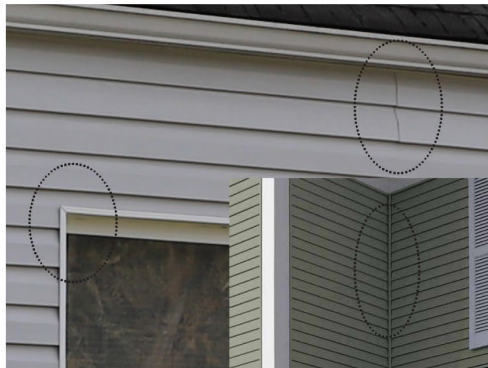
Vinyl siding , look for double vertical joints, vinyl trim around windows, doors and inner corners locking siding ends in place, or soffits enclosed with vinyl.
